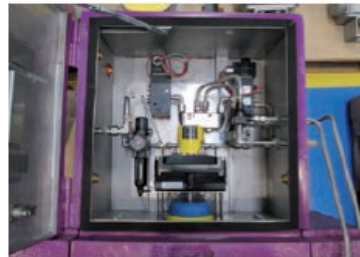
K-CAB HOUSING: CONTROL SET PROTECTION
